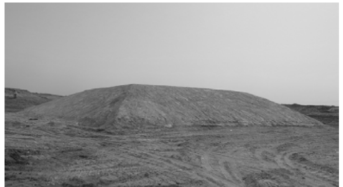
Figure 5. Picture of trial embankment
