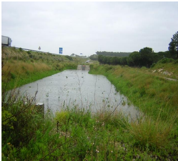
Figure 5. Photos of the retention pond during surface TDR measurements and 9 hours after the rainfall began
