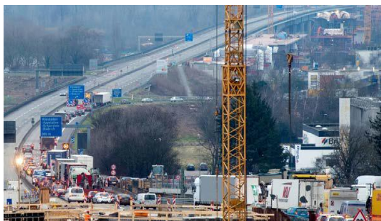
Picture 3. Existing bridge with new construction in progress (Samstag & Stremmel, 2016)
