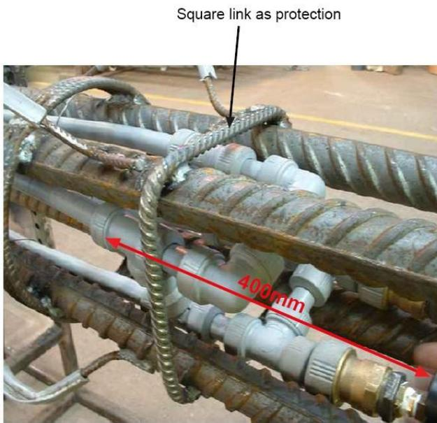
Figure 2.3 CFA pile cage and geothermal pipe, from Arup (2005)
