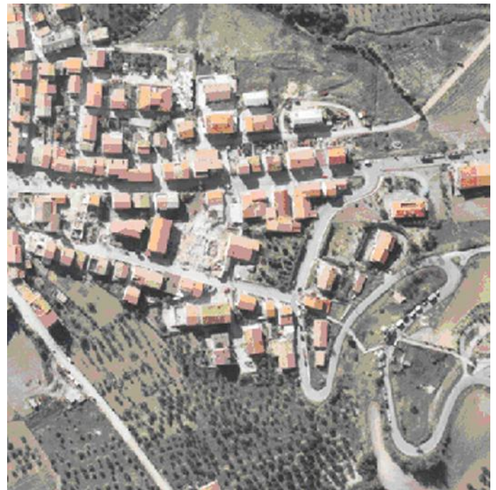
Figure 1. Aerial view of San Giuliano's school after earthquake.
