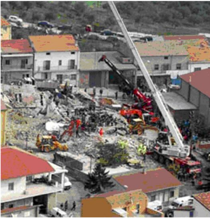
Figure 2. View of collapsed school.
