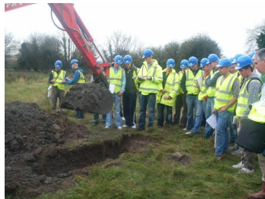
Figure 3: Students logging trial pits and recovering bulk samples
