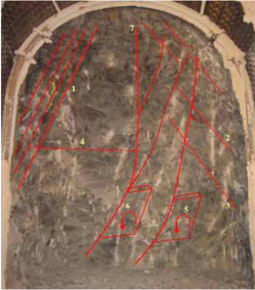
Figure 4. Aspect of the fault zone as observed in the exploratory adit.
