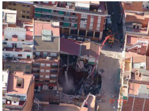
(b) Surface collapse
