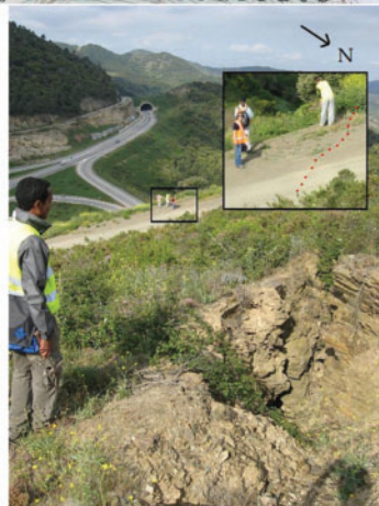
Figure 2. Tacking failure surfaces at Col de la Teixeta, Spain.
