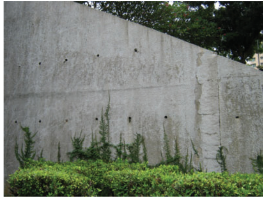
Figure 4. Photograph of a reinforced concrete cantilever retaining wall in campus taken by a student.
