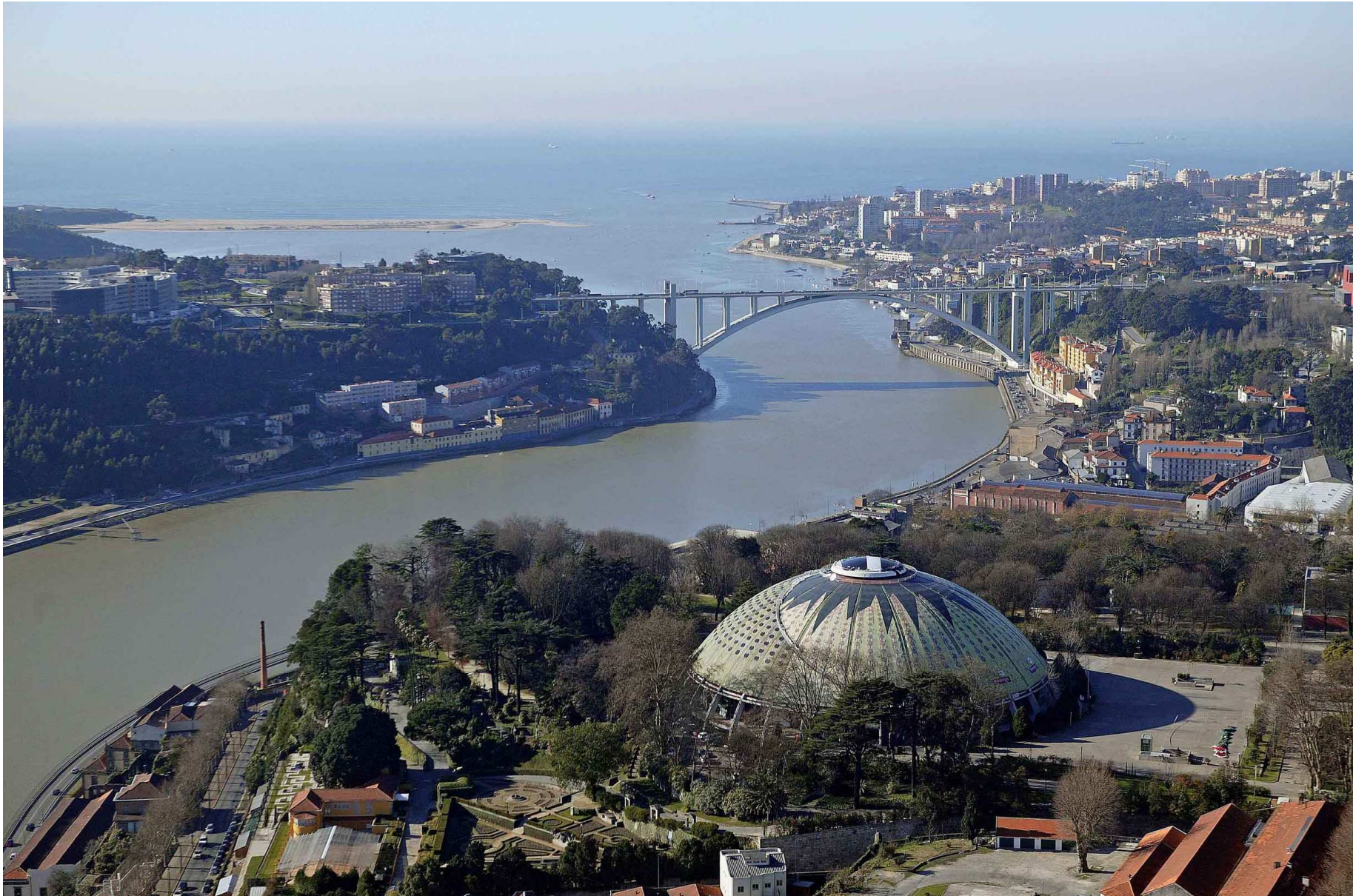
Arrábida Bridge, the largest reinforced concrete arch in the world at the date of its conclusion, Edgar Cardoso, 1963
