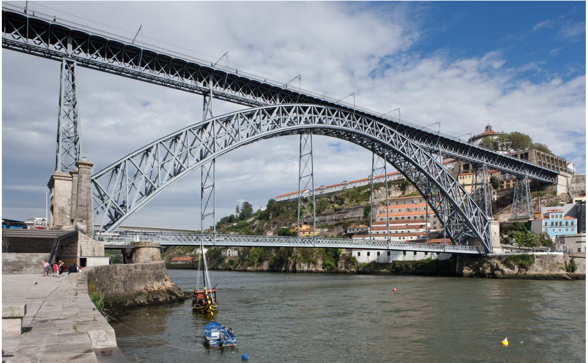
Luíz I Bridge, the unique XIX century iron bridge with two decks in the world, T. Seyrig, 1886
