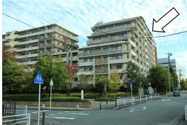
Figure 1. Subsided building in Yokohama
