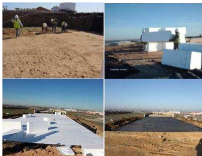
Fig. 7 Construction of EPS Geofoam
