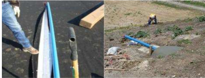
Fig. 8 Horizontal inclinometers installation
