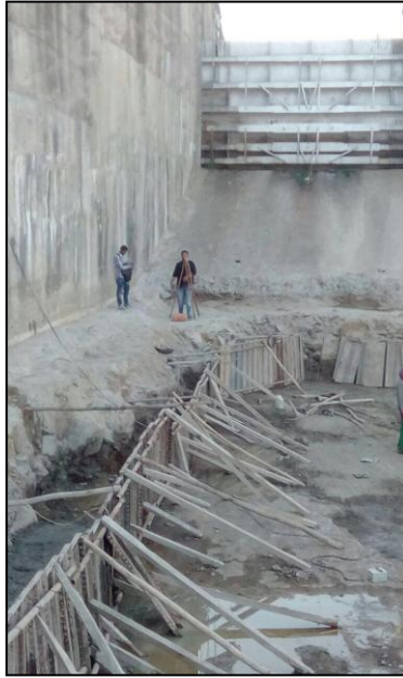
Photo – 3 Construction of Cut-off under Abutment
