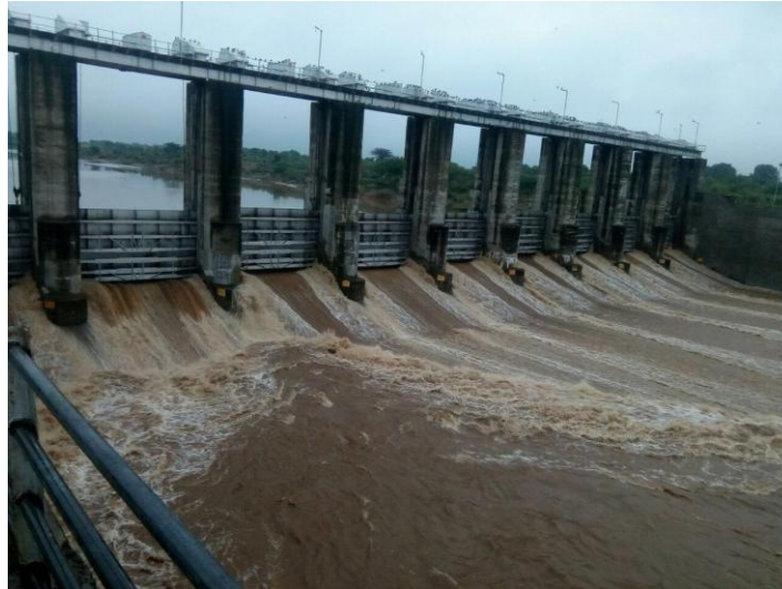
Photo – 5 Post-Repair Performance of Dam
