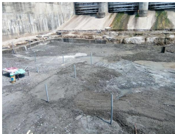
Photo – 4 Construction of Peripheral Cut-off
