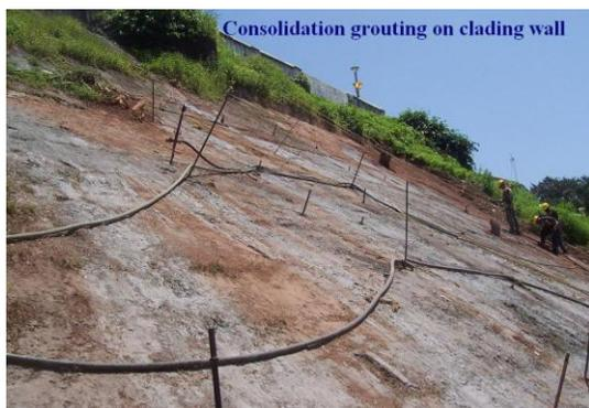
**Figure 6 Grouting over the cladding wall**
