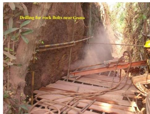
**Figure 7 Drilling for Rock bolting**
