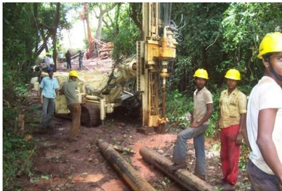
**Figure 11 Vertical piling in progress**
