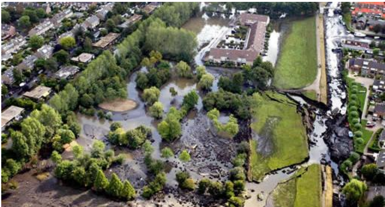
Figure 3. Aerial view of the dike breach at Wilnis
