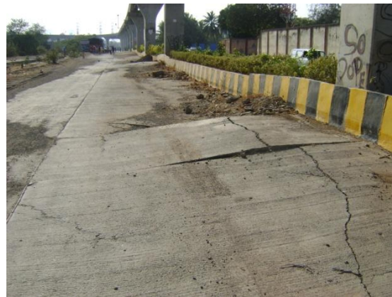
Figure 2b Distress in PQC slabs around Monorail pillars (Sion-Koliwada Road)
