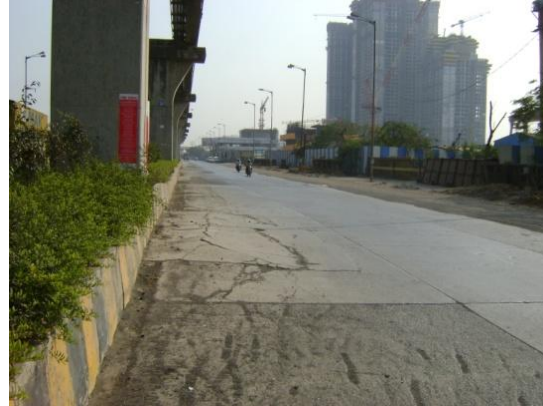
Figure 2a Distress and Cracking of PQC slabs around Monorail pillars (Anik-Wadala Road)
