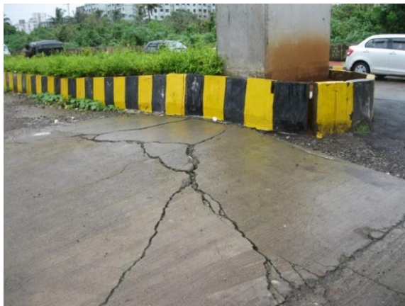
Figure 2b Distress in PQC slabs around Monorail pillars (Sion-Koliwada Road)
