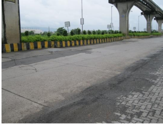
Figure 2a Distress and Cracking of PQC slabs around Monorail pillars (Anik-Wadala Road)
