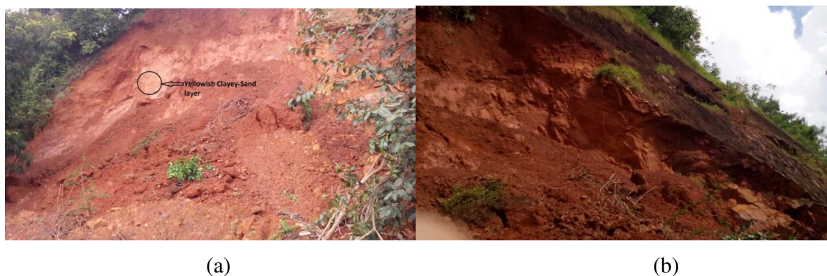
Figure 4: (a) Photo showing yellowish clayey sandy layer, (b) Photo showing failure of slope.
