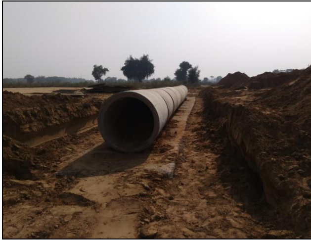
Figure 4(a) Laying of Hume pipe culvert
