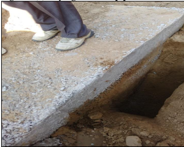
Figure 4(c) casting of raft for Hume pipe culvert
