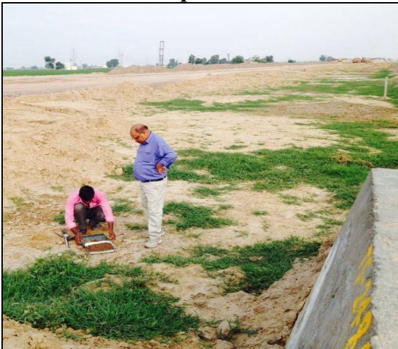
Fig 5(c) In situ density measurement using sand replacement method
