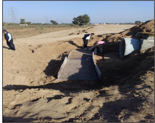
Figure 4(b) casting of raft for head wall
