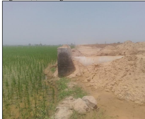
Figure 4(d) Casting of head wall
