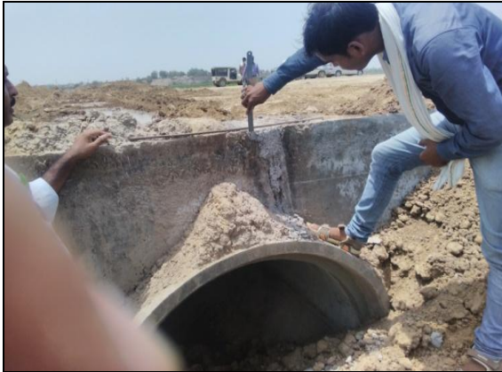
Fig 5(a) Measurement of settlement of head wall and comparison with RLs
