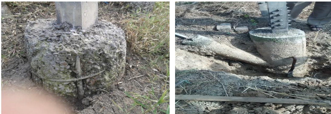
Figure 3. Present condition of the in-service piles
