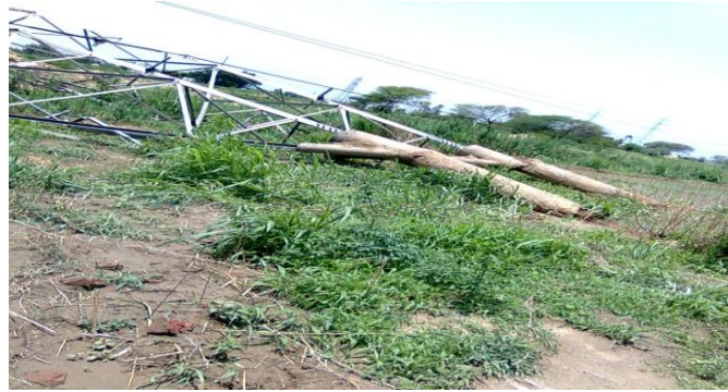
Figure 1. Uprooted pile foundation with tower
