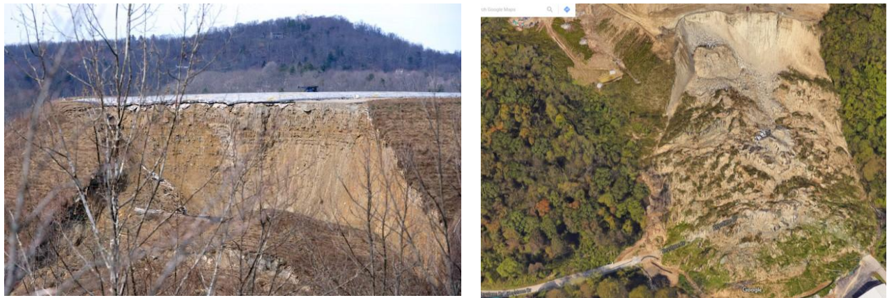
Figure 2. The failure of Yeager airport expansion runway as reported by Charleston Gazette-Mail on 12 Mar 2015
