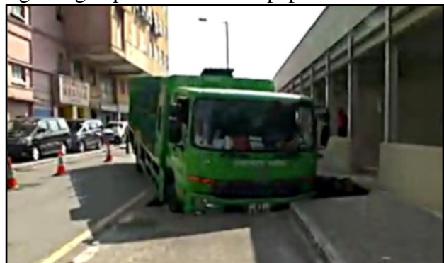
Figure 2. Falling of a drinking water delivery truck into a sinkhole.
