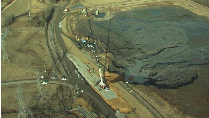
**Figure 2: Coal ash spill at Dan River due to stormwater pipe collapse
