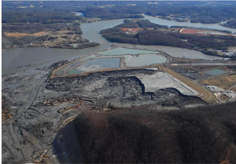
**Figure 1: Failure of the dike causing coal ash spill at Kingston fossil plant (Source: TVA, 2011)**
