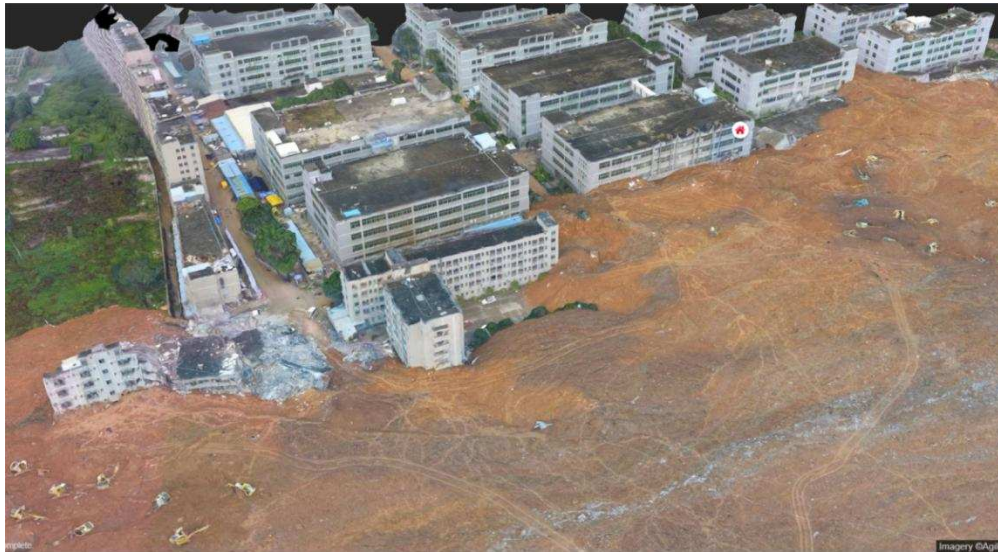
Figure. 3. Buildings that faced the landslide.
