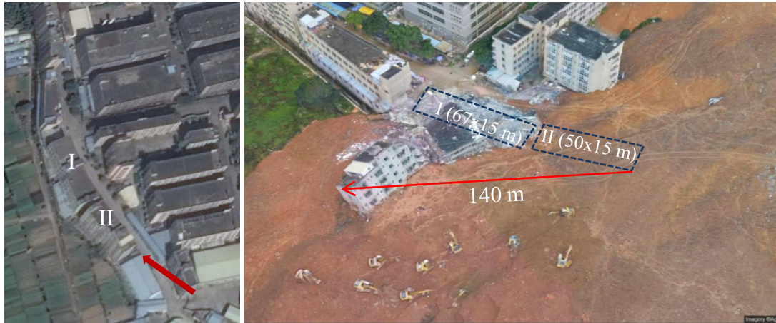
FIG. 10. Front view of the building that was subject to sliding and overturning failure. (3D images with permission from Prof. Quan Long, https://www.altizure.com/project/567791fe9e0bd5b06ced19ba/model ).
