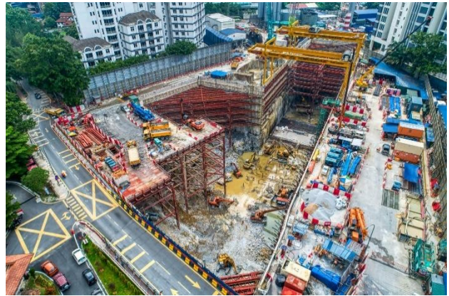
Figure 9. Conlay Station at final excavation level (Courtesy of MMC-Gamuda)
