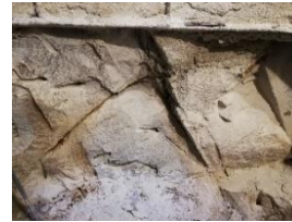
Figure 4. Typical caisson shaft surface in rock socket
