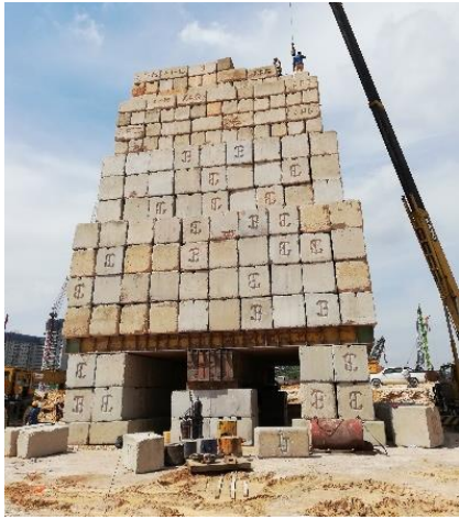
Figure 2. Static load test set-up system with kentledge blocks
