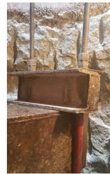
Figure 13b. Connection of reinforcement bar
