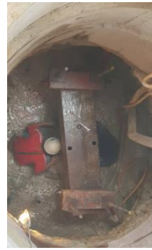
Figure 13a. Load test set-up inside hand-dug caisson
