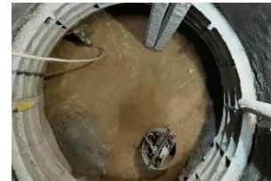
Figure 5. Caisson pile base condition after proper cleaning
