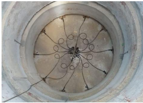
Figure 7. Caisson shaft load test set-up with 10 nos. of hydraulic jack
