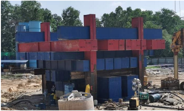
Figure 3. Reaction frame system for a 6000-tonne static load test
