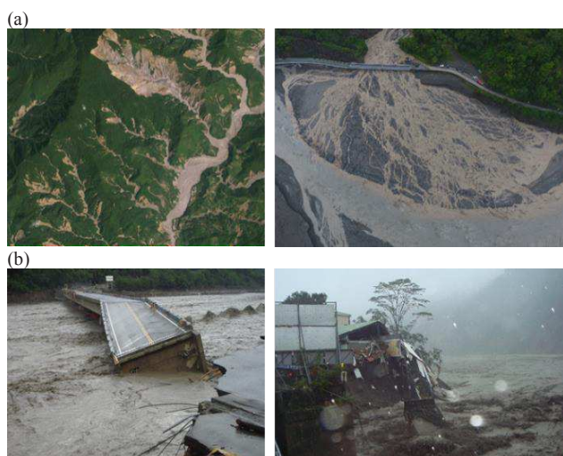
Figure 2. Figure 2-(a) shows the massive landslides and debris flow alluvial fans directly impacted the road built along the river, Figure 2-(b) shows in facing compound disasters, rehabilitation construction became quite difficult and hard to maintain.
