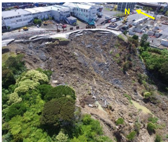
Figure 3. Aerial oblique photograph of landslide headscarp taken 7 January 2018.
