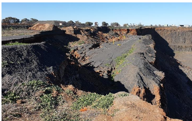
Figure 6. The eastern high wall following occurrence of the failure. The deep shadow to the right of the picture is the high wall into the pit, and the deep shadow to the left is the back scarp of the failure. The grey material in the middle of the photograph is the asphalt of the now inaccessible access road.
