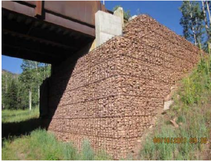
Figure 1: Typical MSE structure (bridge abutment) at the Colony Project.
