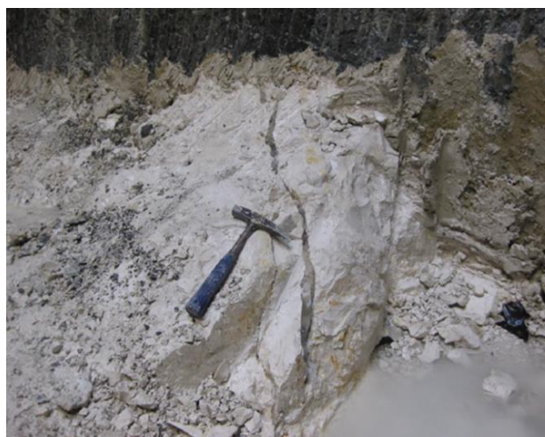
Figure 6. Grouted fissure exposed during the shaft excavation (photo by Tim Newman).
