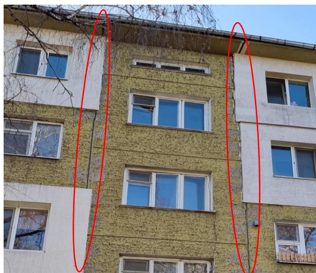
Figure 11. Cracks on the facade of a building in Sofia.
