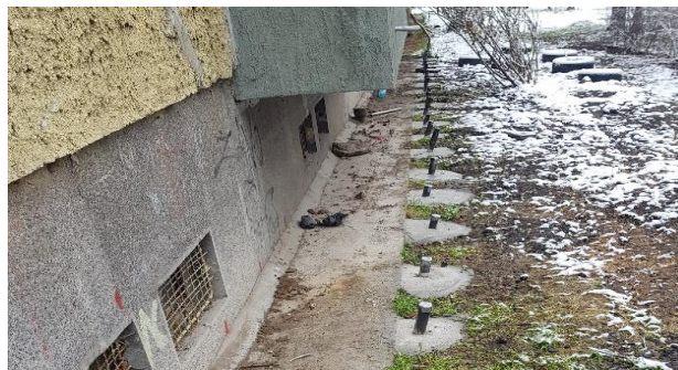
Figure 12. Reinforcement of the soil under the strip foundations by the TAM grouting method along the entire perimeter of the building.
