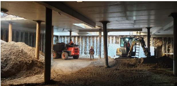
Figure 7. Excavation for foundation slab
