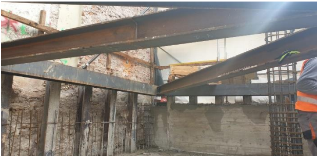
Figure 5. Steel structure used for propping
