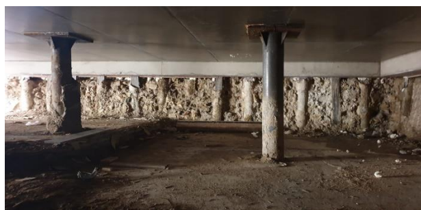
Figure 4. Piles \Phi 300 mm and \Phi 400 mm
