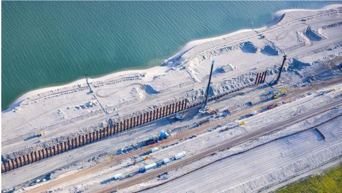
Figure 5. Tubular pile installation at Amaliahaven in the port of Rotterdam
