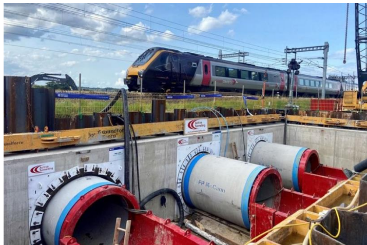
Figure 5: Launch Pit, during operation of railway
