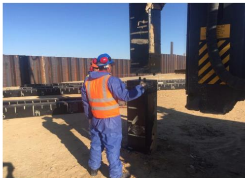
Figure 1. Installation of precast concrete joint pile
