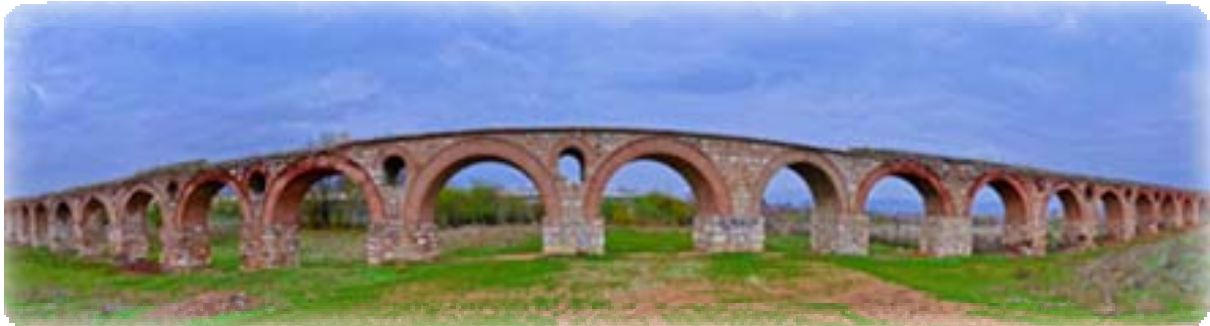
Figure 3. Panoramic view of the Aqueduct in Skopje
