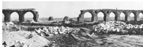
Figure 2. Aqueduct after the dynamites' exercise
