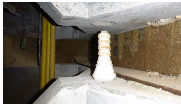
Figure 15: Disconnection of sheeting dowels
