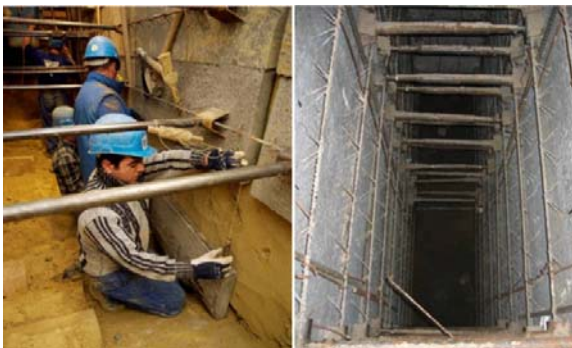
Figure 1: Deep braced excavation by hand
