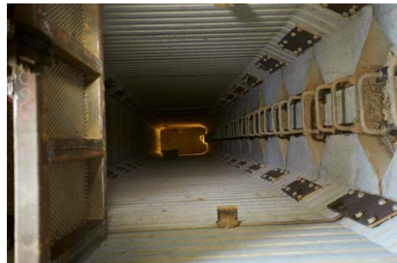
Figure 16: Final result of T1, top view
