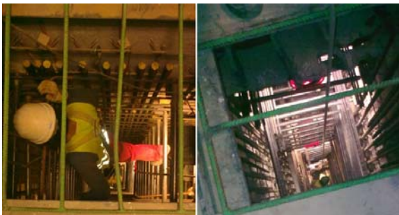
Figure 2: Rebarred trenches
