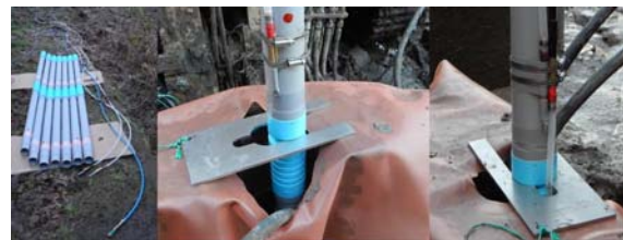
Figure 12. Left – part of 3D measuring casing with uncoiled FBG chains, center – lower end of the chain fitted to the casing, right – connection of two FBG chains, after (Záleský et al. 2014)
