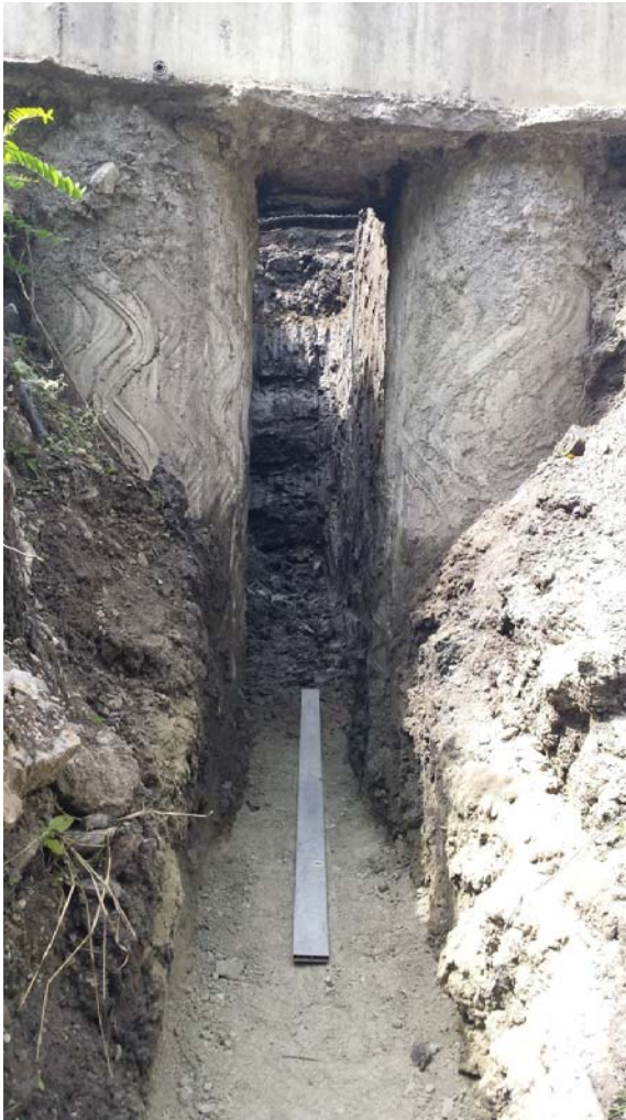
Figure 10. Photo of performed piles during drainage installation
