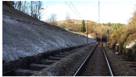
Figure 10. Photo of renewed stone facing with pile retaining wall
