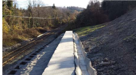
Figure 11. Photo of performed pile retaining wall
