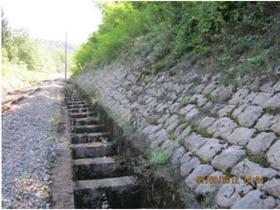
Figure 1. Previous solution – drainage channel and stone facing
