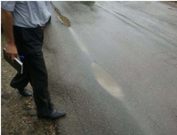
Figure 1.b. Differentiated settlements resulted from poor compaction works
