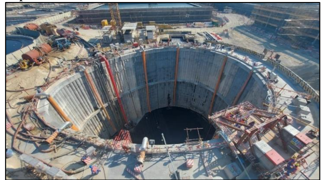
Figure 12. Secant pile wall after completion of excavation
