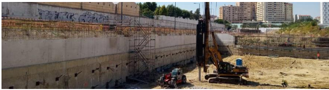
Figure 5. Pile Driving Analyser preliminary tests being executed at lot 2
