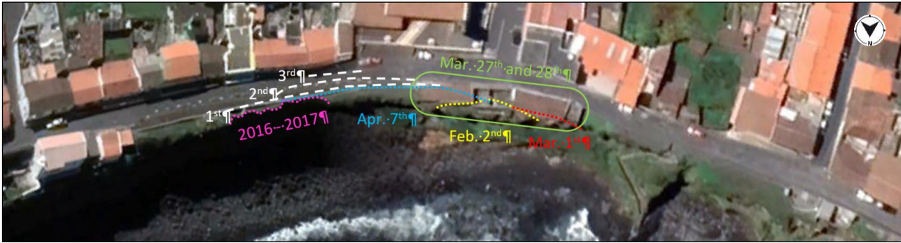
Figure 2. Affected areas on the Calhetas cliff: the alignment of existing cracks (dashed), the unstabilised areas (dotted) and the demarcation of demolished buildings / those affected by this crisis (continuous). Google Earth image (June 2022).
