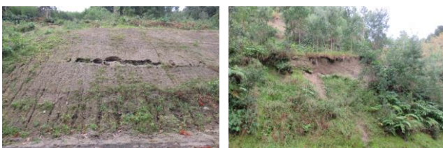
Figure 4. Site n°. 4 - Erosion on the slope face (on the left). Geomorphological instability at site no. 6 (on the right).
