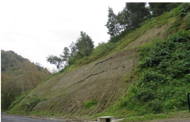
Figure 3. Site no. 4 - Slope re-profiling.
