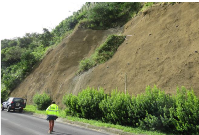
Figure 8. Site no. 14 - Application of nailing, metal mesh and shotcrete.
