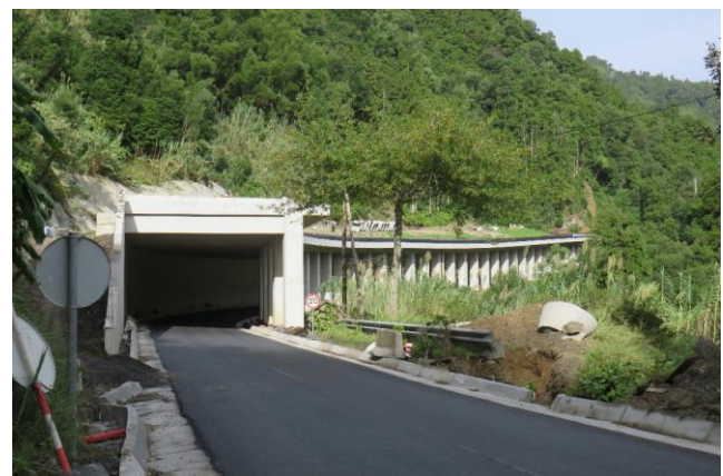
Figure 6. Site no. 12 – Semi-tunnel.
