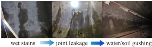
Figure 1. Leakage defects in shield tunnels.
