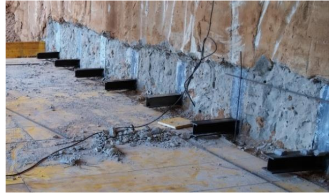
Figure 5. Photo of the HEA sections for connecting the slab at "Largo do Ambiente".
