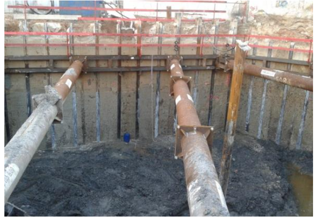
Figure 10. Photo of the "May Flower" construction site before the application of the second level of bracing.
