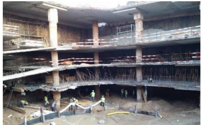
Figure 11. Photo of the execution of the fifth and final slab band at "Largo do Ambiente".
