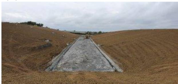
Figure 3. Heave Trial at formation level.
