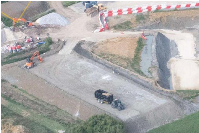
Figure 4. Lime Stabilised Glacial Till Trial in Newton Purcell,
