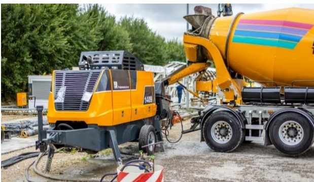
Figure 17. Concrete supply via concrete pump.
