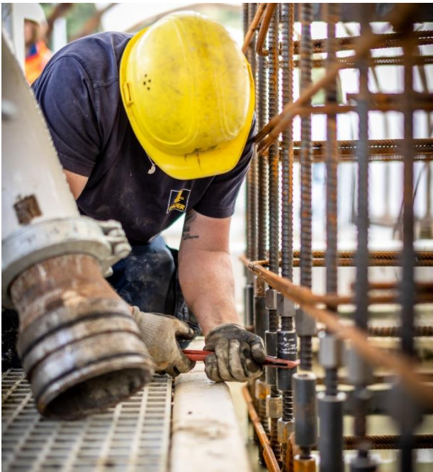
Figure 16. Cage coupling.
