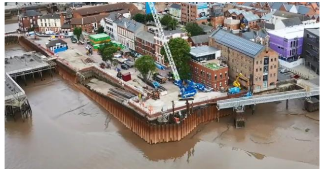
Figure 3. Construction works at Victoria Pier.
