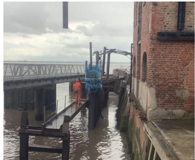
Figure 6. Installation of pressed piles along the River Hull.
