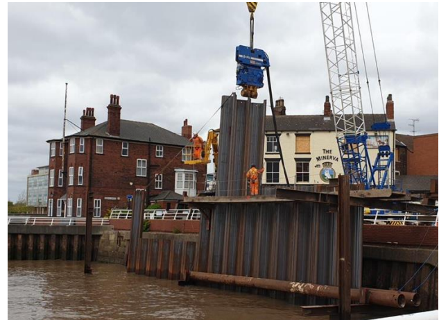
Figure 5. Installation of raked piles along the Humber.
