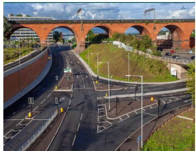
Figure 1. Image of the New Link Road looking towards the Stockport Viaduct, with the M60 to the south.
